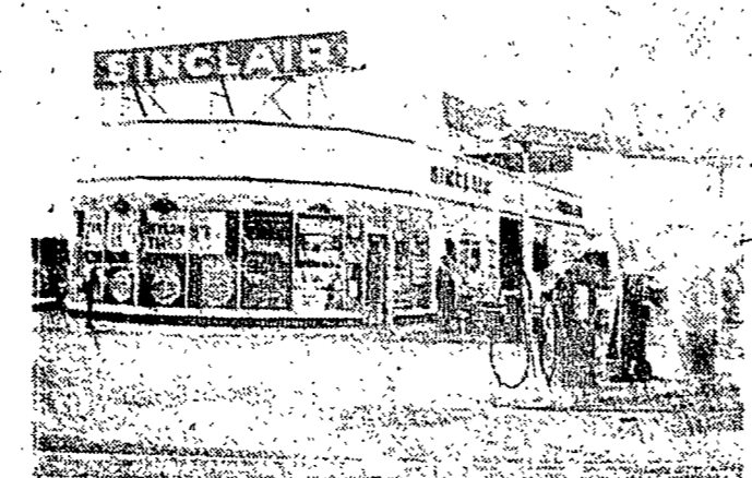
FLOREST SERVICE STATION 7970 Milwaukee
