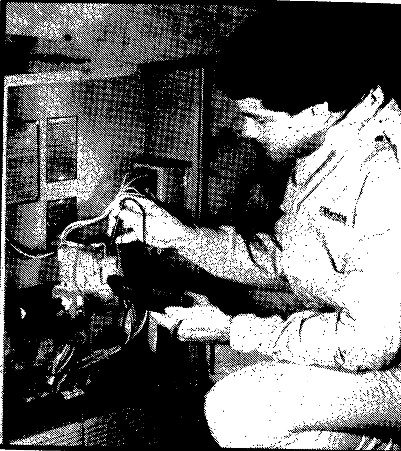
A pre-season boiler inspection includes electronic ignition testing.
