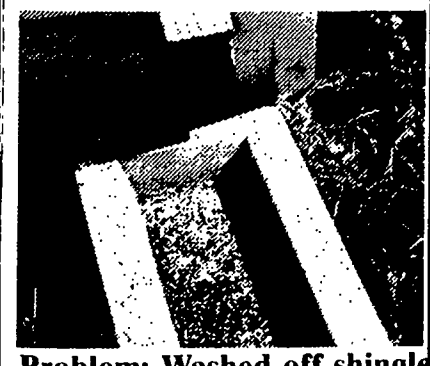
Problem: Washed-off shingle granules.
