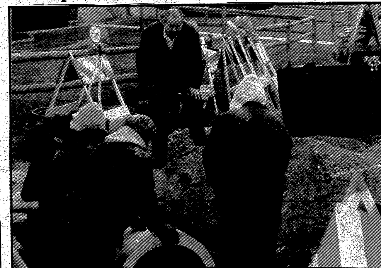
Maine Township Highway Commissioner Bill Fraser supervises a highway department crew as they lay new storm sewers to replace broken conduits on roads in unincorporated Maine Township. The repair work is an ongoing project to maintain the storm sewer system in good working condition.
