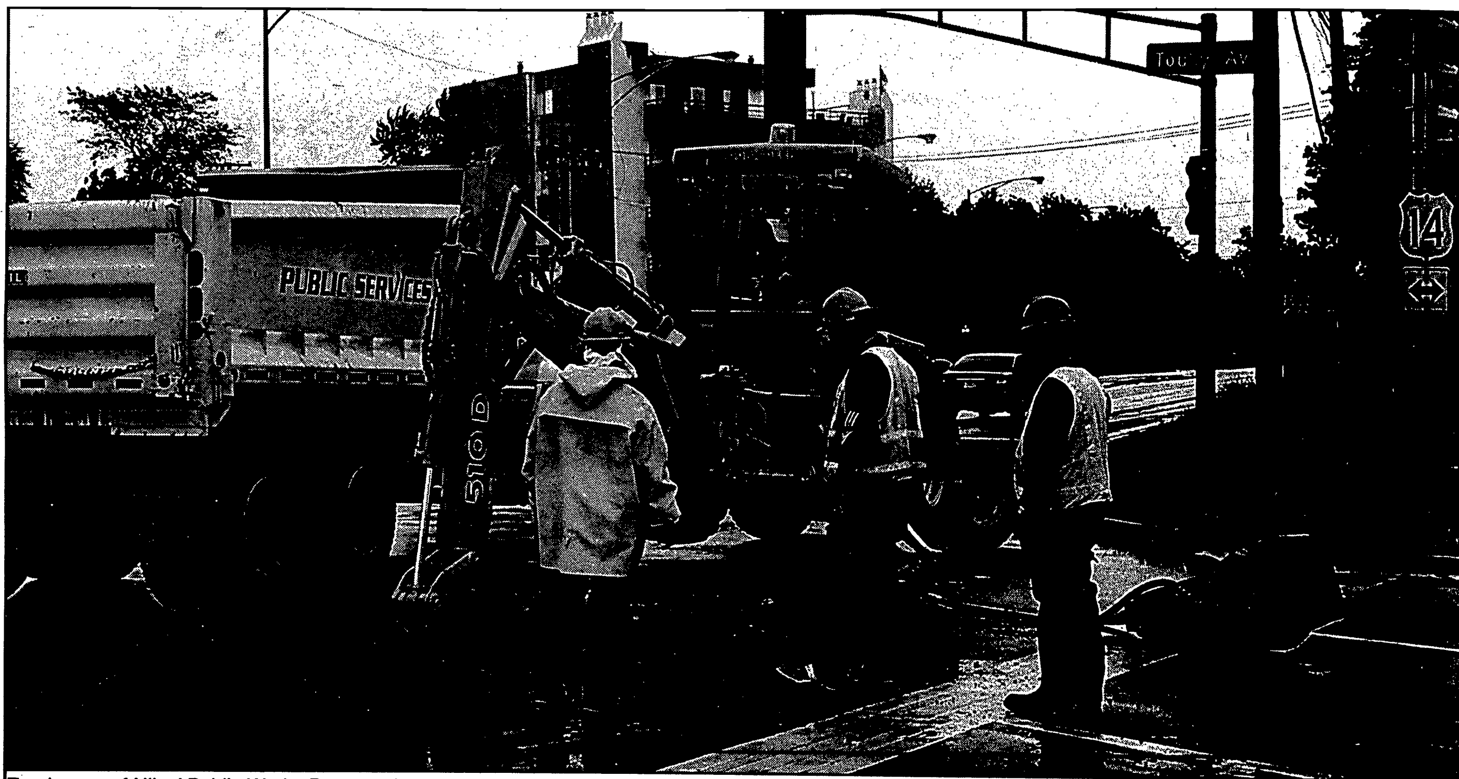
Employees of Niles' Public Works Dept. work to repair a water main break which left 150 homes without water Monday, Sept. 1.
