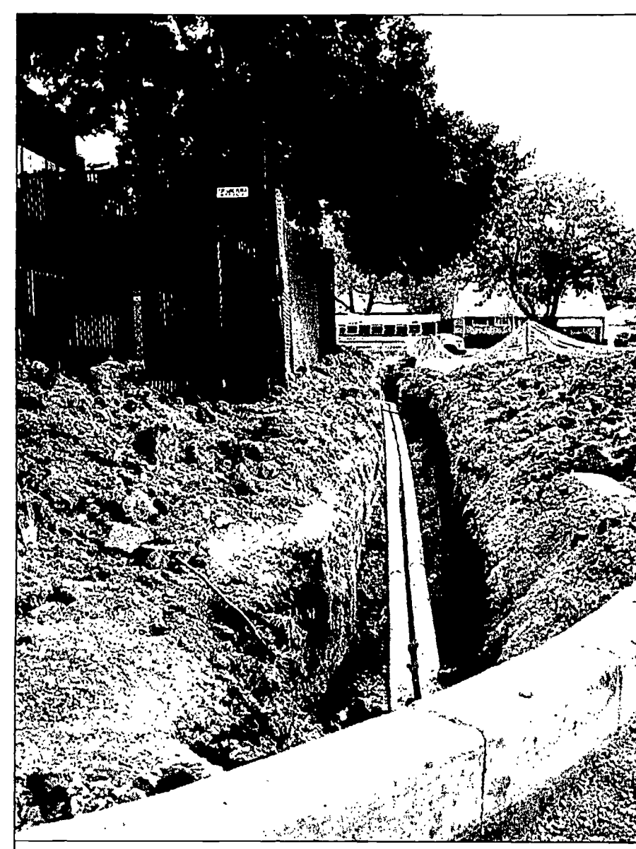
A trench was recently dug around the Oasis Water Park Building in order to route telecommunications lines to a new cell tower being constructed to resemble a flag pole at the southwest corner of the Niles Park District's property.
