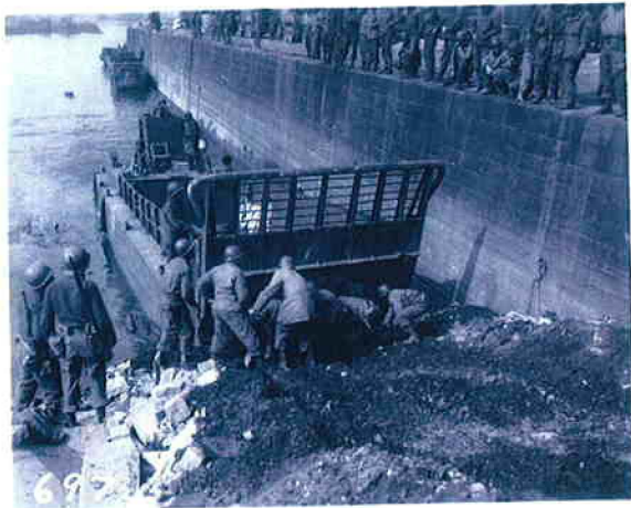
Engineers working on approaches for LCMs
