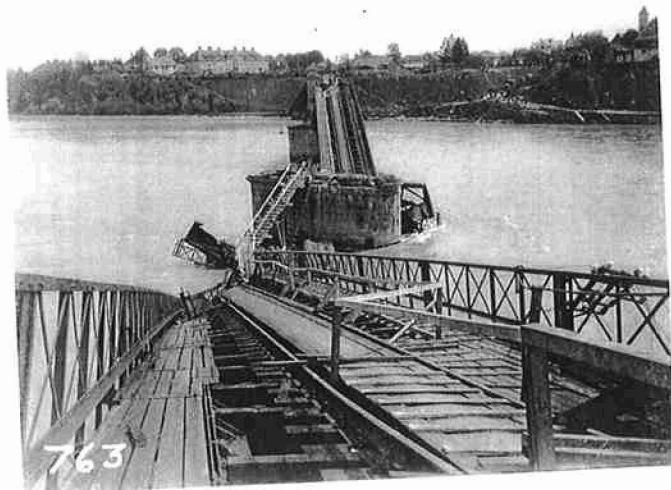
Blown bridge made passable
